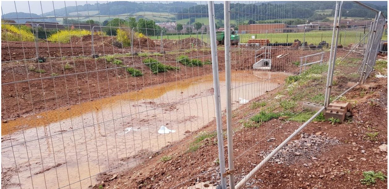
Raising the level of the site with spoil from the industrial land.
